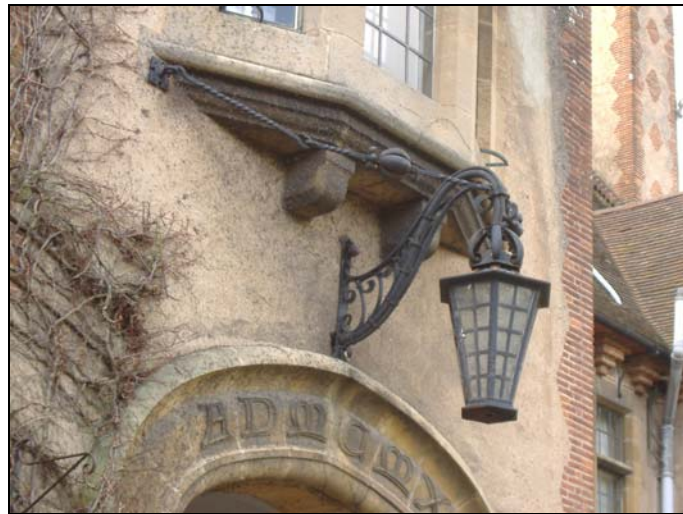
The original lamp over the front door
