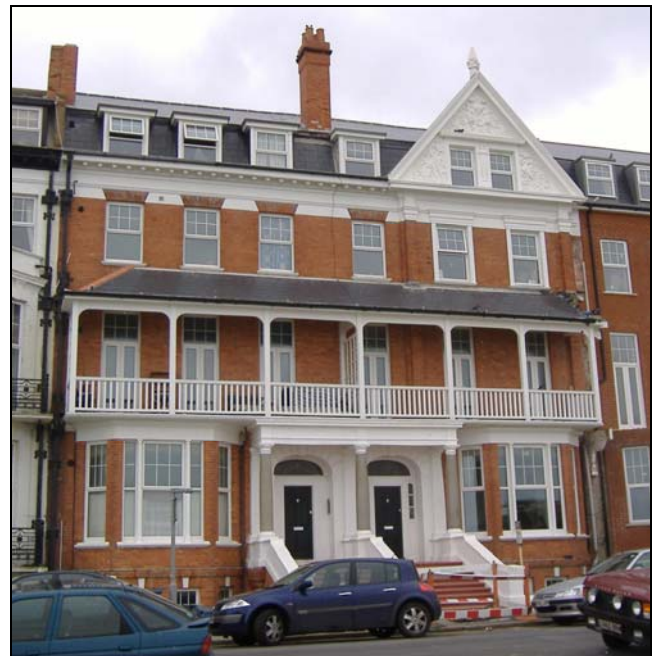
Nos 4 & 5 Lewis Crescent, Cliftonville – now converted to housing
