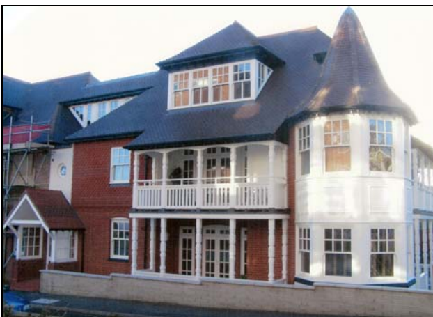
The large extension to the rear of No 19 Sea Road, Westgate-on-Sea. This excellent extension has incorporated all the features of the existing building and fits extremely well into Westgate
