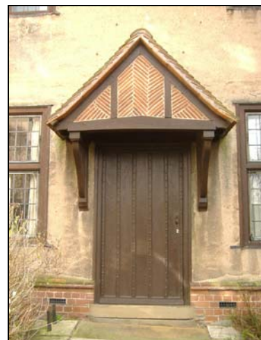
Door into garden at rear of house
